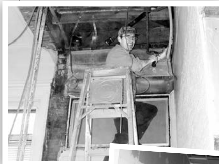
Administration Building Renovations in progress
