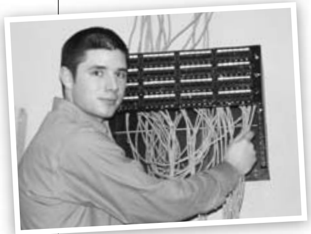
Brent Miles wires the dormitory computer network
